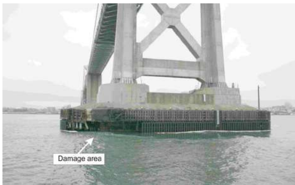
Damaged fendering system at the base of the BayBridge Delta tower.
